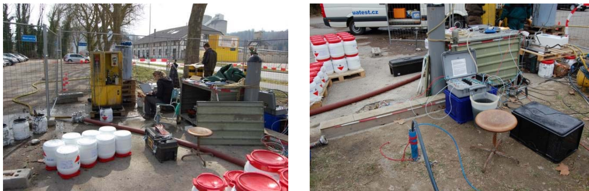
Figure 7: Injection of FerMEG12 (nZVI) into the Solvay site © VEGAS, University of Stuttgart, Germany
