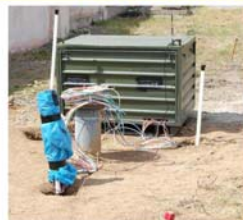
Figure 6. Heads of monitoring arrays for in situ measurement (on Spolchemie pilot site) contracted to measuring hardware in protective box © VEGAS/USTUTT, University of Stuttgart, Germany
