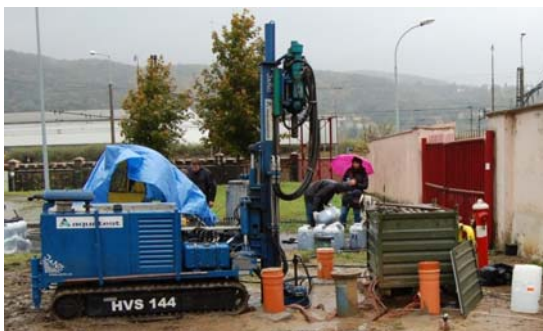
Injection at Spolchemie pilot site 1 (VEGAS/USTUTT)
