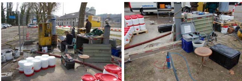
Injection of FerMEG12 (nZVI) into the Solvay site (© VEGAS / University of Stuttgart, DE)
