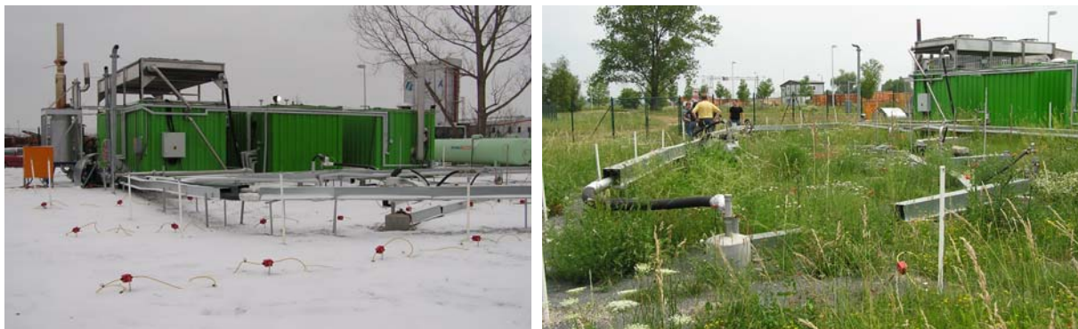
Figure 4: mobile remediation unit (MOSAM) and pilot site
