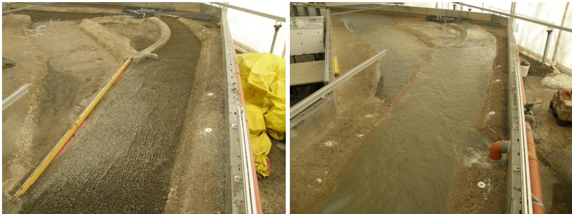
Abb. 10.3: Situation of the inflatable weir before (left) and after (right) the flood wave
