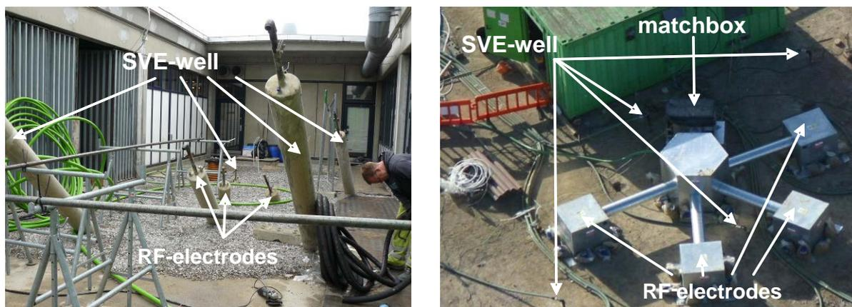
**Figure 3.4: Options of electrode arrangements for the RF-supported soil vapour extraction at different sites (right: protection of the RF electrodes)**
