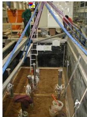
Installation of groundwater drainage pipes
