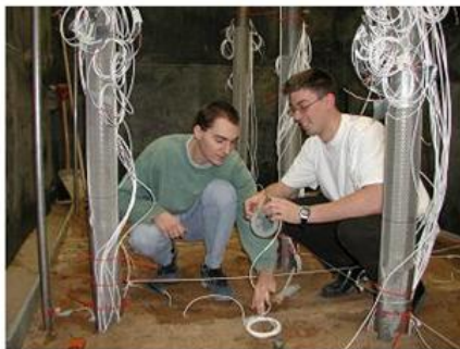
installation of temperature sensors
