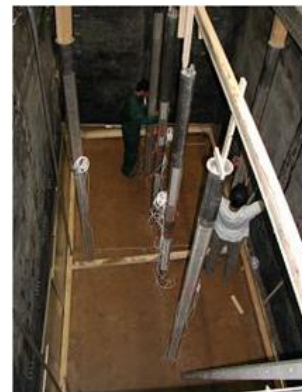
installation of vertical wells
