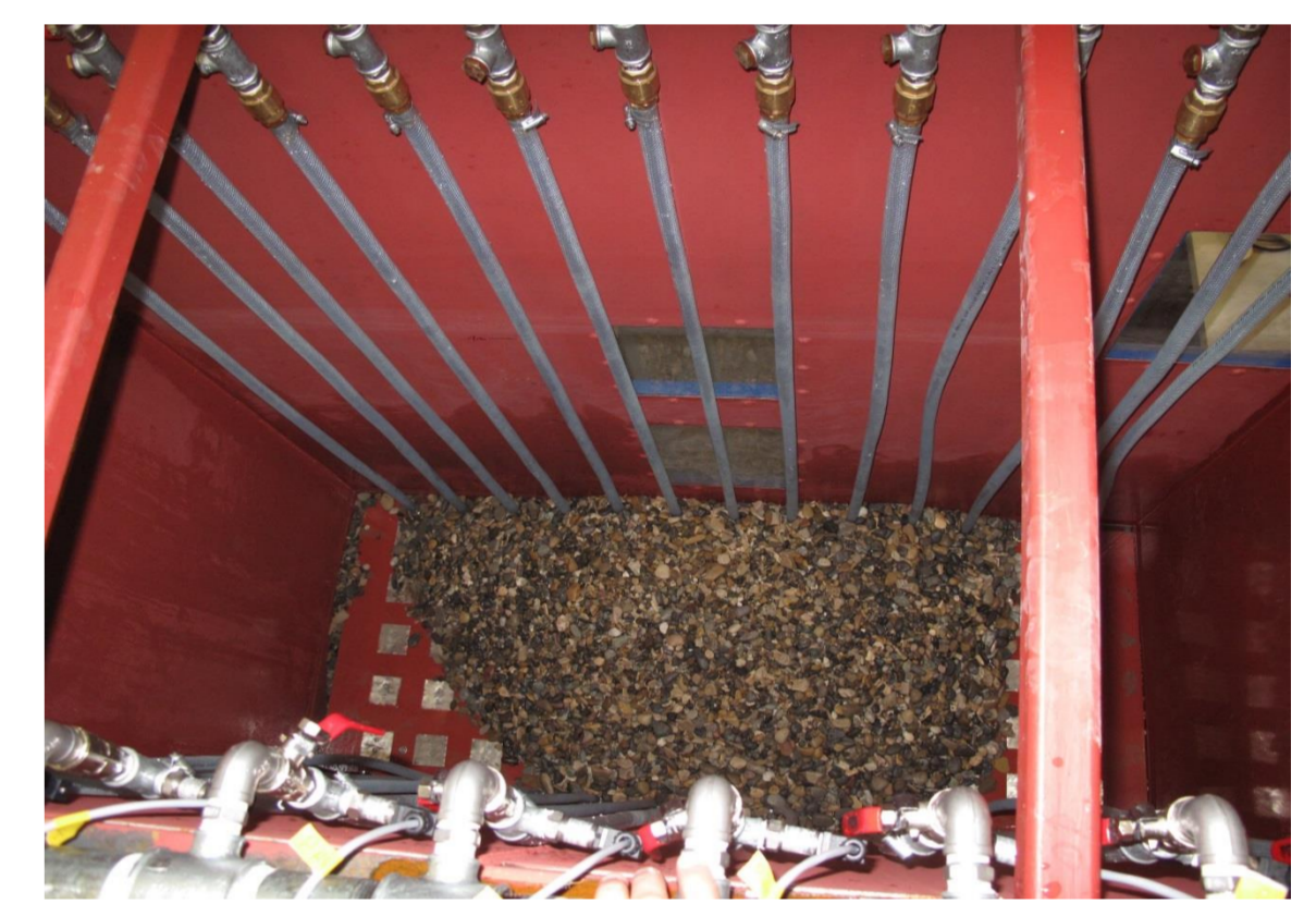
Fig. 4: Introduced coarse cobble mixture on top of the aeration units (plan view)
